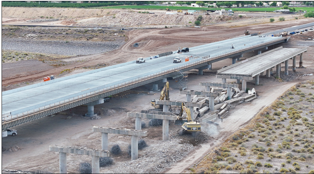
When compared side-by-side, the width of the new bridge is at least double of the original and will provide for additional lanes of travel. Viewpoint looking south towards Mesa. Courtesy of Maricopa Department of Transportation
