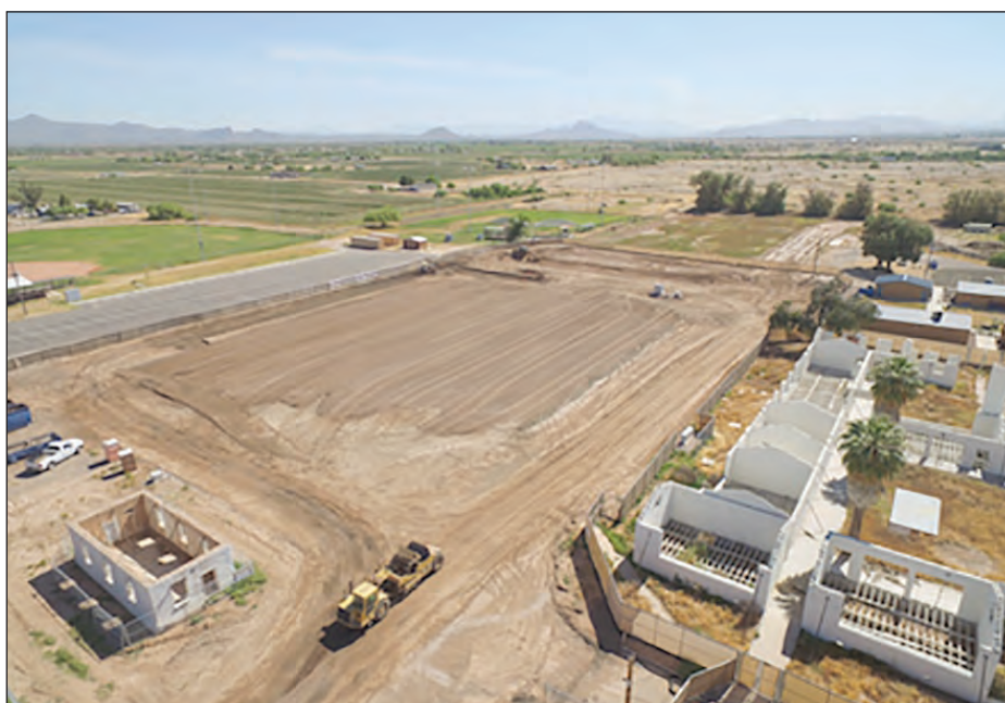
Building pad being constructed.
