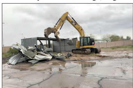
Demolition of BIA Day School Bus Barn.
