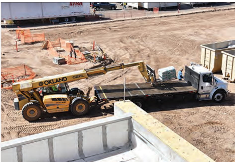
Construction vehicle lifting supplies for crews.
