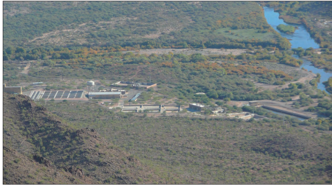
The Verde Water Treatment Plant, off Fort McDowell Road and north of the Granite Reef Diversion Dam, was built in 1948.
