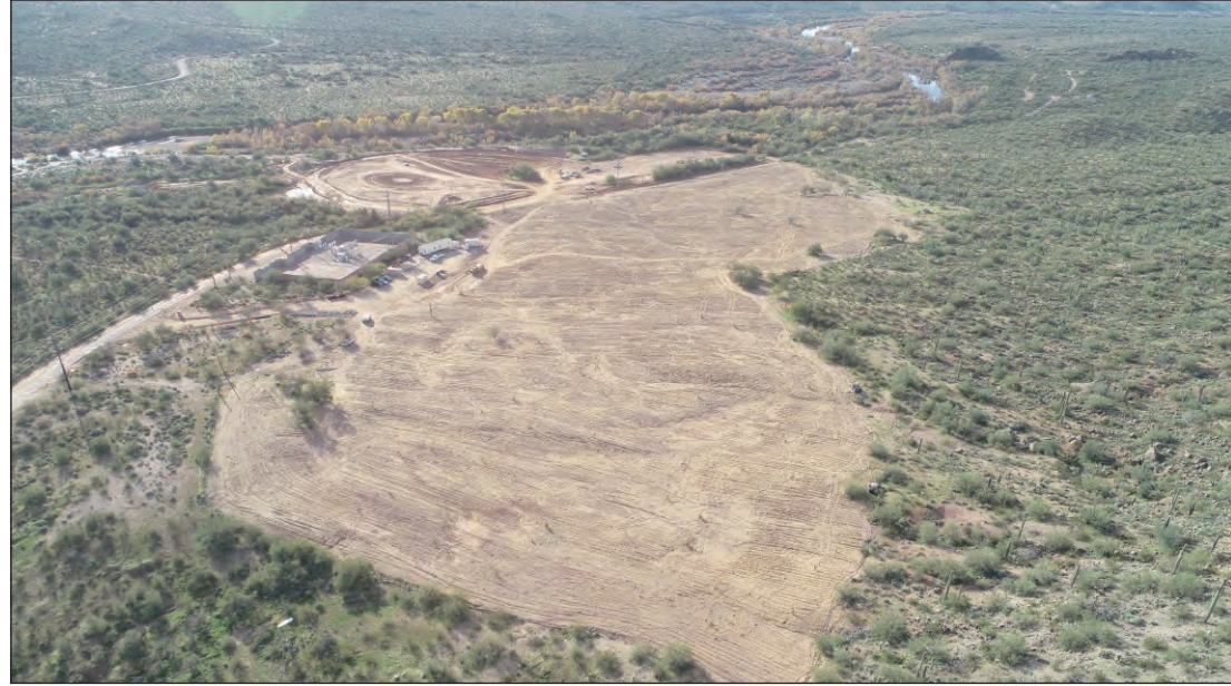
Picture taken after the Verde Water Treatment Plant demolition and clean-up.
