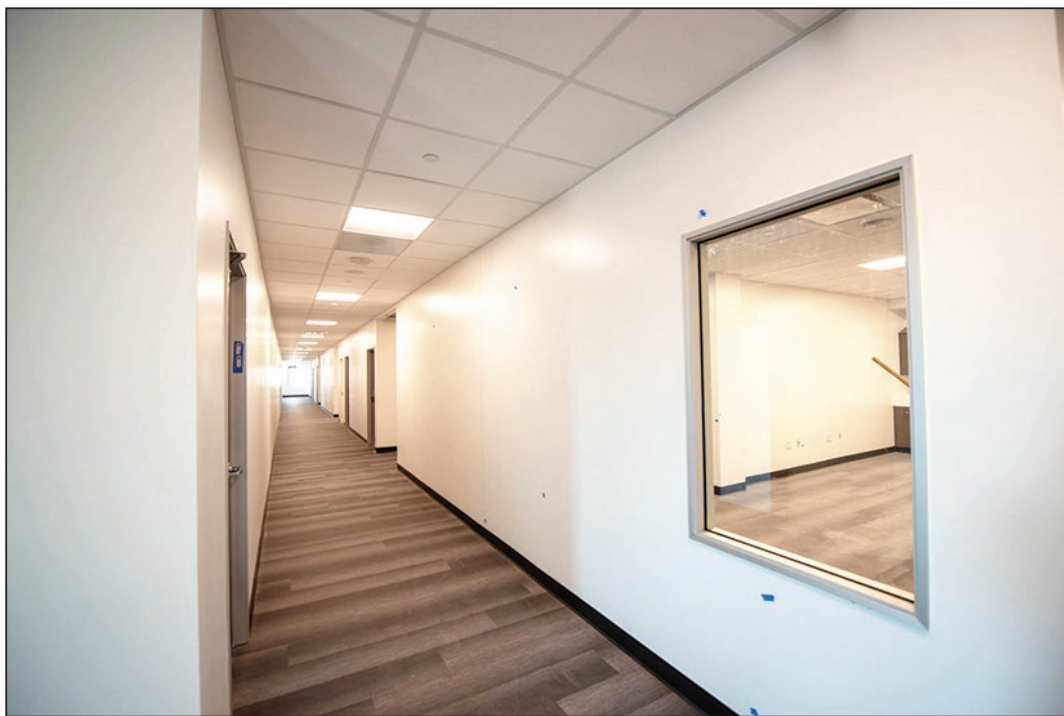
Completed area in primary care, awaiting equipment installation.
