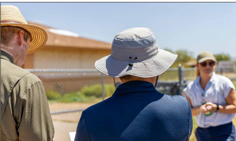
Members from the FEMA Region 9 office conduct a Preliminary Damage Assessment on a house damaged during July's wildest storms. PDA's help tribal communities, like SRPMIC to receive much needed resources, during times of emergency.
