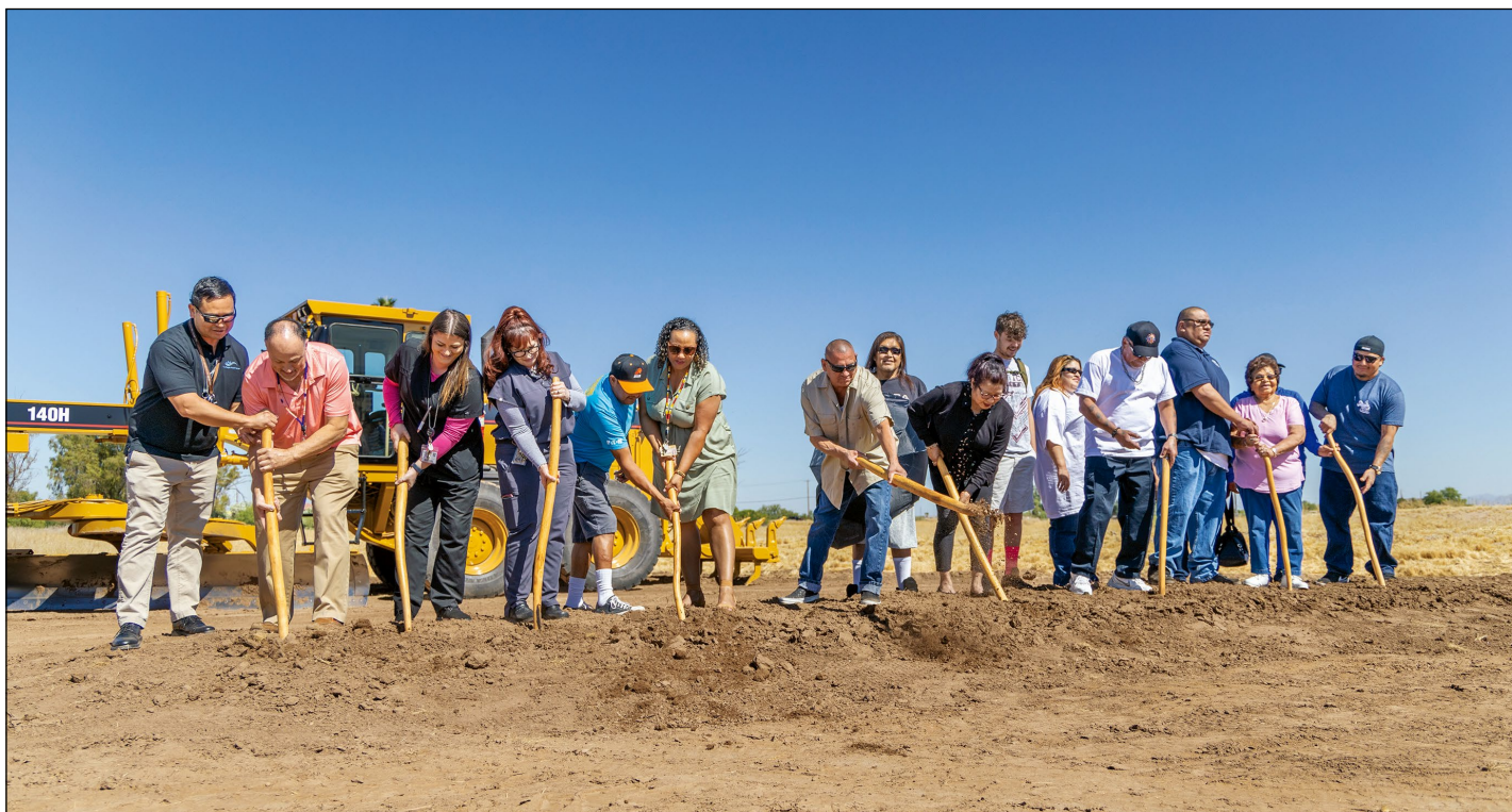
JTR program staff, patients and graduates help break ground on new JTR project site on May 9.
