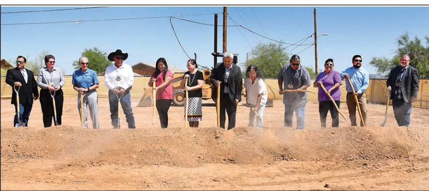
Councilmembers, Community partners and departments break ground with shovels in hand at the Lonely Cactus Expansion Rentals site on May 3.
