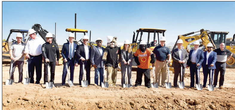
Banner Sports Medicine breaks ground on their new facility in the SRPMIC Pima Corridor.
