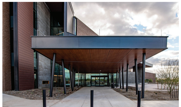
The columns in the front entrance are skewed to recall the mesquite poles of traditional ramadas.
