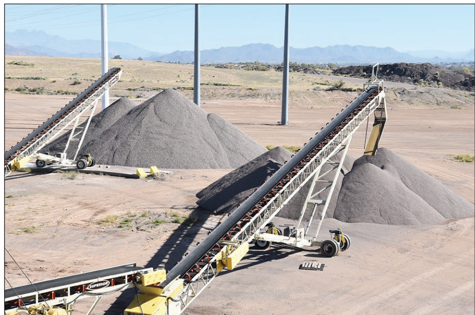
The final stage of the process, where refined aggregate is unloaded using a feed conveyor belt.
