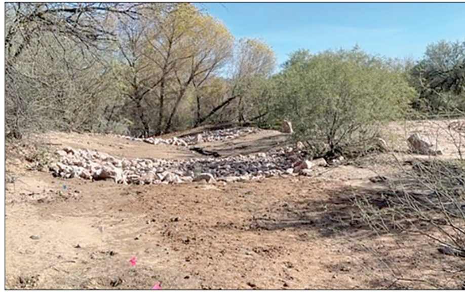
Arroyo site after construction.
