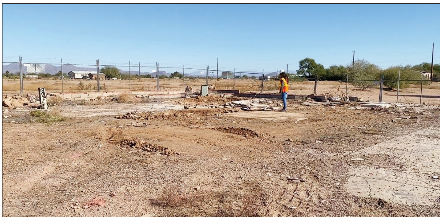
Northwest corner of the Roadrunner Lake Resort Site. Senior environmental specialist- Brownfields- Lily Bermejo looking at are where potholing was conducted while searching for asbestos. Photos courtesy of Lily Bermejo
